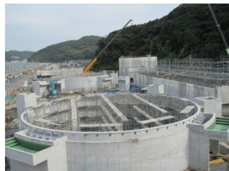
Onshore fish tank of 20 m in diameter to be used for bluefin-tuna-rearing experiments (under construction)
