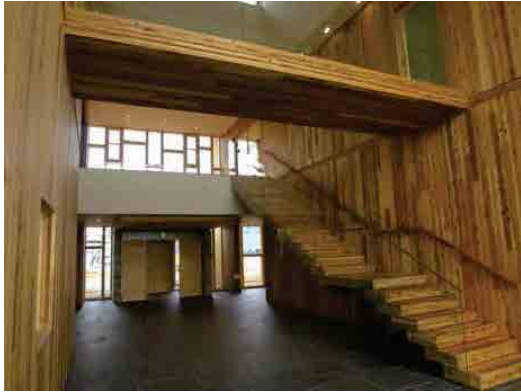
Photo ii: Building using CLT (Kochi prefecture)
