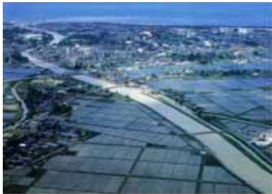
(国営施工)幹線排水路
