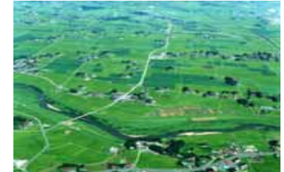
(県営施工)ほ場整備
