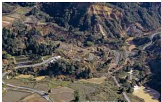
A landslide on farmland following the Mid-Niigata Prefecture Earthquake
