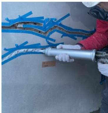
ひび割れ補修工
