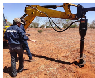
Excavation of planting holes using construction machinery
