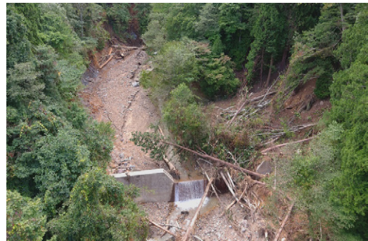
Control of sediment and driftwood runoff by forest conservation facilities (Kazamaura village, Aomori Prefecture)
