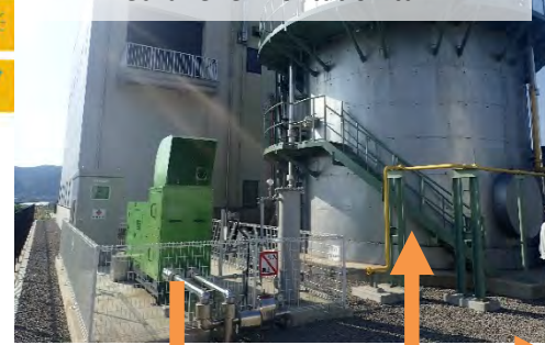
Surplus heat from the gas power generation equipment is used to dry methane digestion sludge
