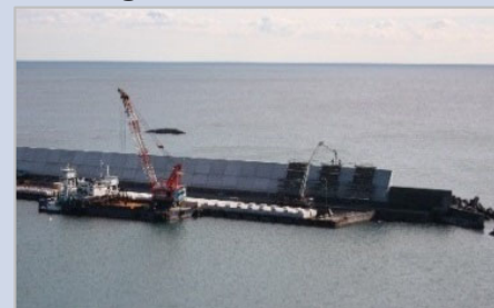
Raising of breakwaters
