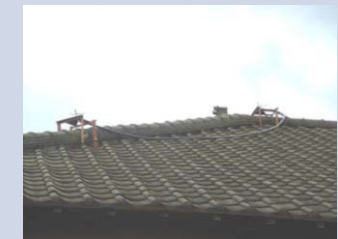
Sprinkler installation on barn roof
