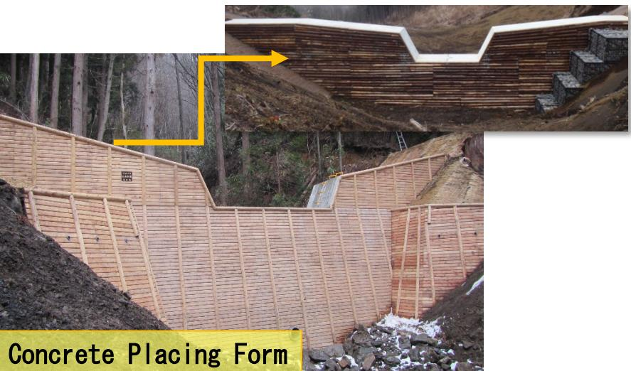
Concrete Placing Form
