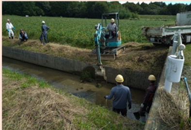
Dredging up mud by members of the organization and employees of a construction company
