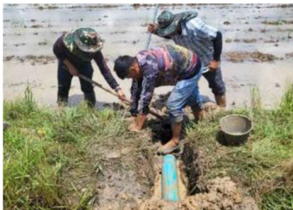
Installation of underground drainage on farmland
