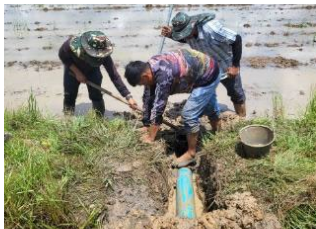
Installation of underground drainage on farmland
