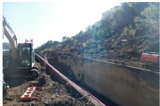
[洪水吐急流水路付近]
