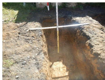
(p) 模擬農道床掘深さ検測 ( H=1.0\text{m} )
