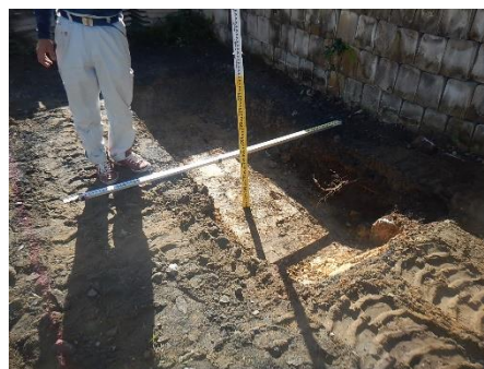
(j) 模擬畑掘削深さ検測 (H=0.4m)
