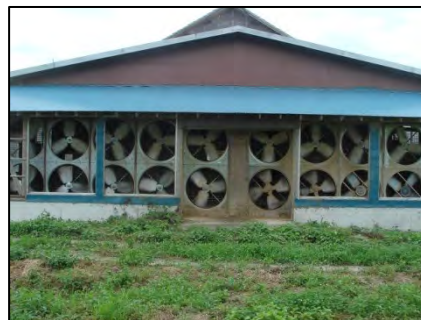
↑牛舎壁面の換気扇
