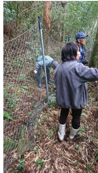
侵入防護柵の点検
