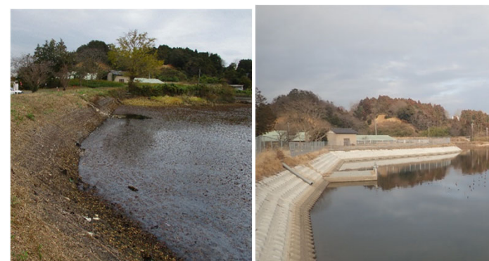
Reservoir embankment before and after elevation construction work Source: Ibaraki Prefecture
