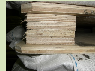
2) Pallets made of plywood
