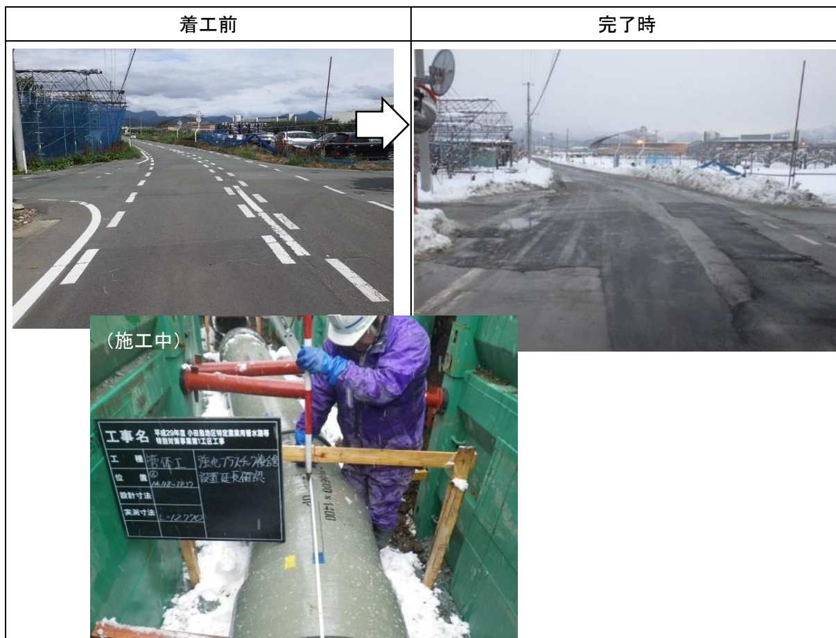
[送水管布設状況 (FRPM 管直径 600mm)]
